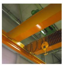
Power supply of the crab on an overhead bridge crane
